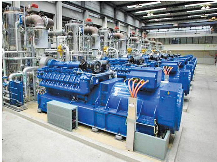
Construction of 2 CHP power plants with a capacity of 33 MW and a solar unit with a capacity of 7.5 MW
